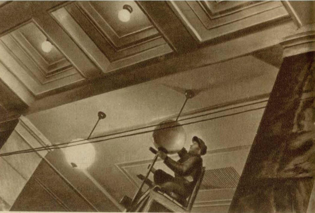
Installing the electric lighting
