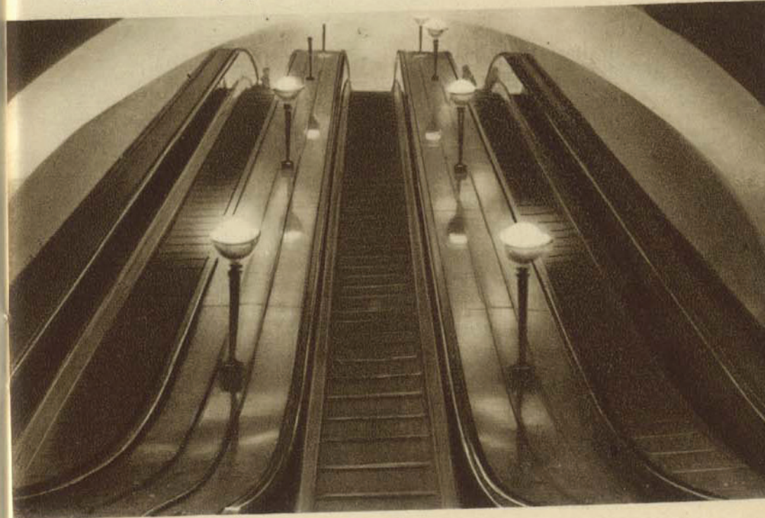
Escalators at Okhotny Ryad
